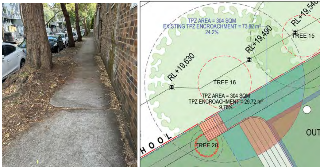
Figures 80 & 81: The proximity of Tree 16 to the existing building edge depicting the lifted paving (Left - Source: Austin 2 nd November 2023) and the floor plan depicting the existing building in the blue hatched line with the proposed building TPZ encroachments shown in pink, batter in blue and scaffold from level 1 and above shown in hatch (Source: General Floor Plan, by Plus Architects, drawing number PLA-PP -1000 dated 15/1/2024). See appendix for larger plans.
