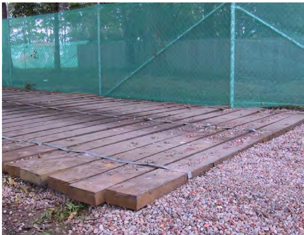
Figure 90- Where access is required through an identified tree protection zone the ground surface shall be protected through appropriate boarding and mulch or gravel placed above the existing ground surface to protect the roots and limit soil compaction. (Photo: Arterra)
